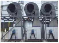
**CENTRIKLON** The compact, high capacity CDS Centriklon centrifugal separator removes dust and chaff even more efficiently than the Clean Air Control system. No moving parts means minimal maintenance.
